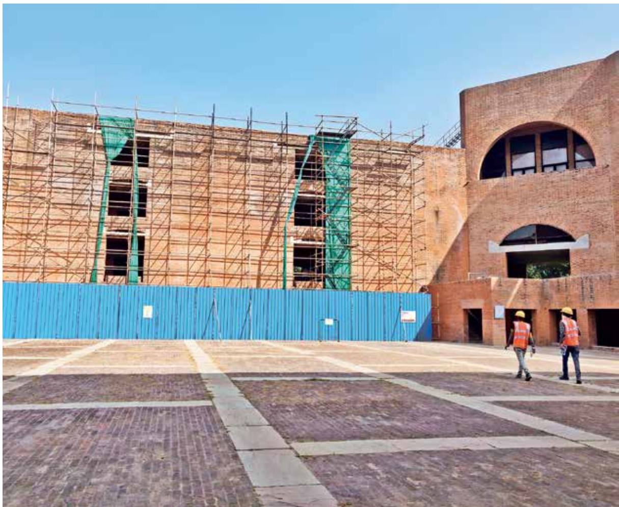
Ongoing restoration of the faculty block in the Heritage Campus
